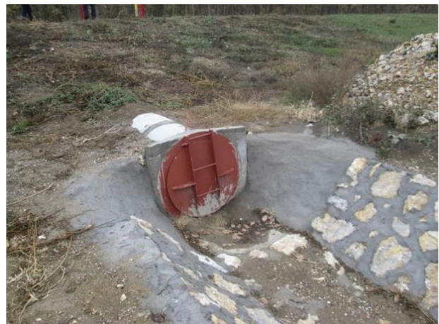
Figure 17: water pipe culvert
